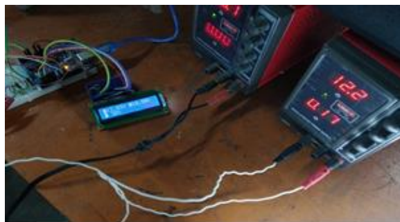
Fig-2: Charge Controller in operation
